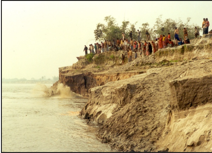
River Bank Erosion
