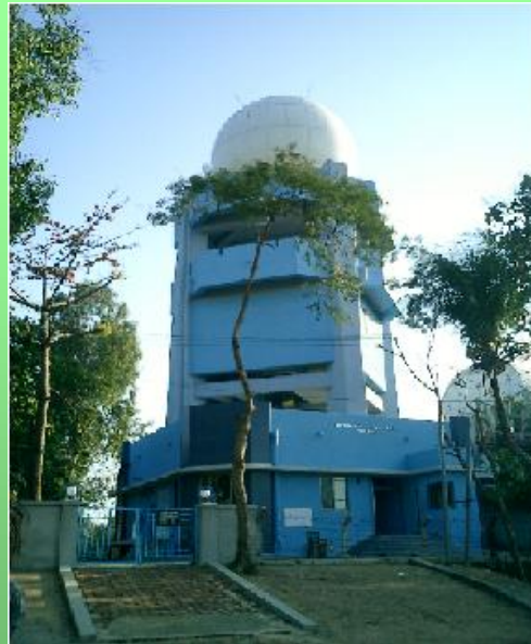
Cox's Bazar Radar
