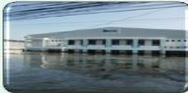
Too Much Water
