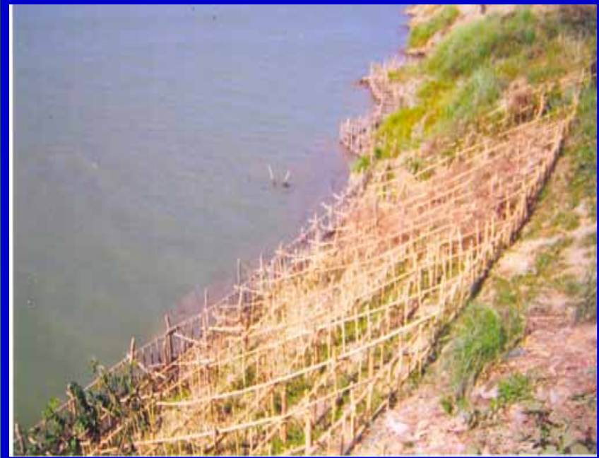
Protection from erosion by using low coast local bamboos.
