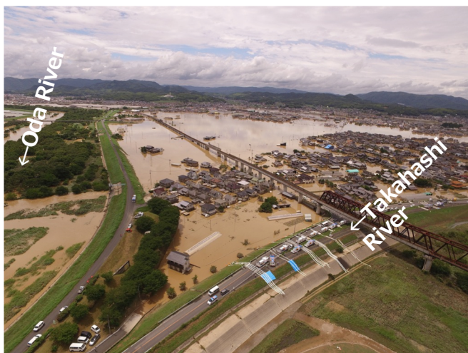
Breached river levee and flooding between Takahashi River and Oda River
