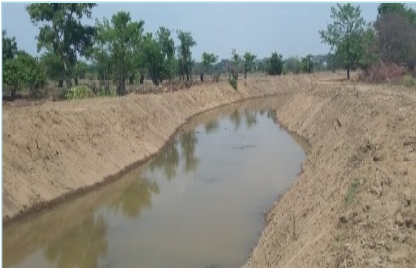
Excavation of Ngabat Yoe Creek
