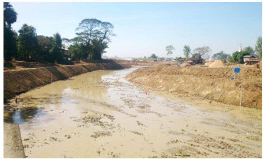
Excavation of Kali Creek
