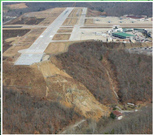
2015 landslide at airport runway
