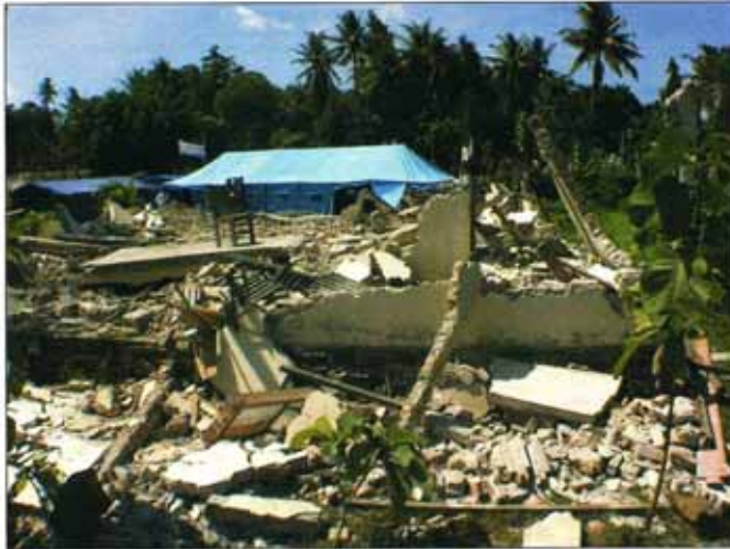
Fig. 1. Collapsed junior high school building in Bantut, south of Yogyakarta, destroyed by the shaking of the Java earthquake.
